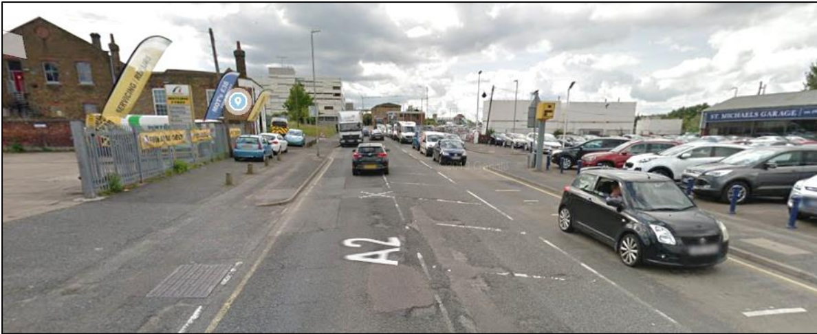
The poor condition of St Michael's Road
